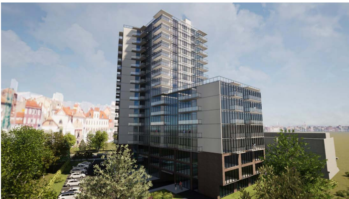
Looking southwest from the rear (northeast) corner of the Subject Site.
