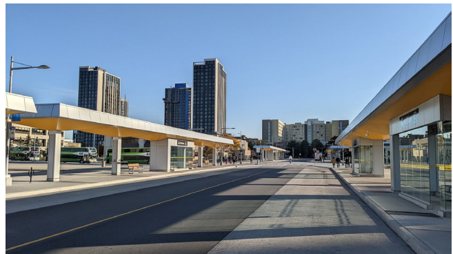
Above: University of Waterloo GRT Station
