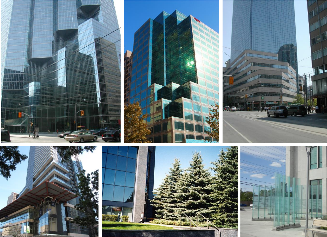
Image 9 – Examples of Wind Control Solutions at Grade: Building Massing Refinements, Canopies and Landscaping/Screens
