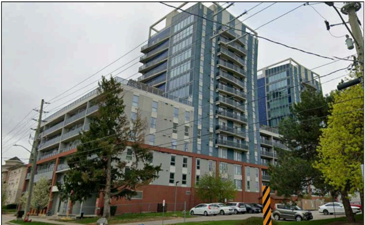
Figure 13 - The Hub Development at 130 Columbia Street West
