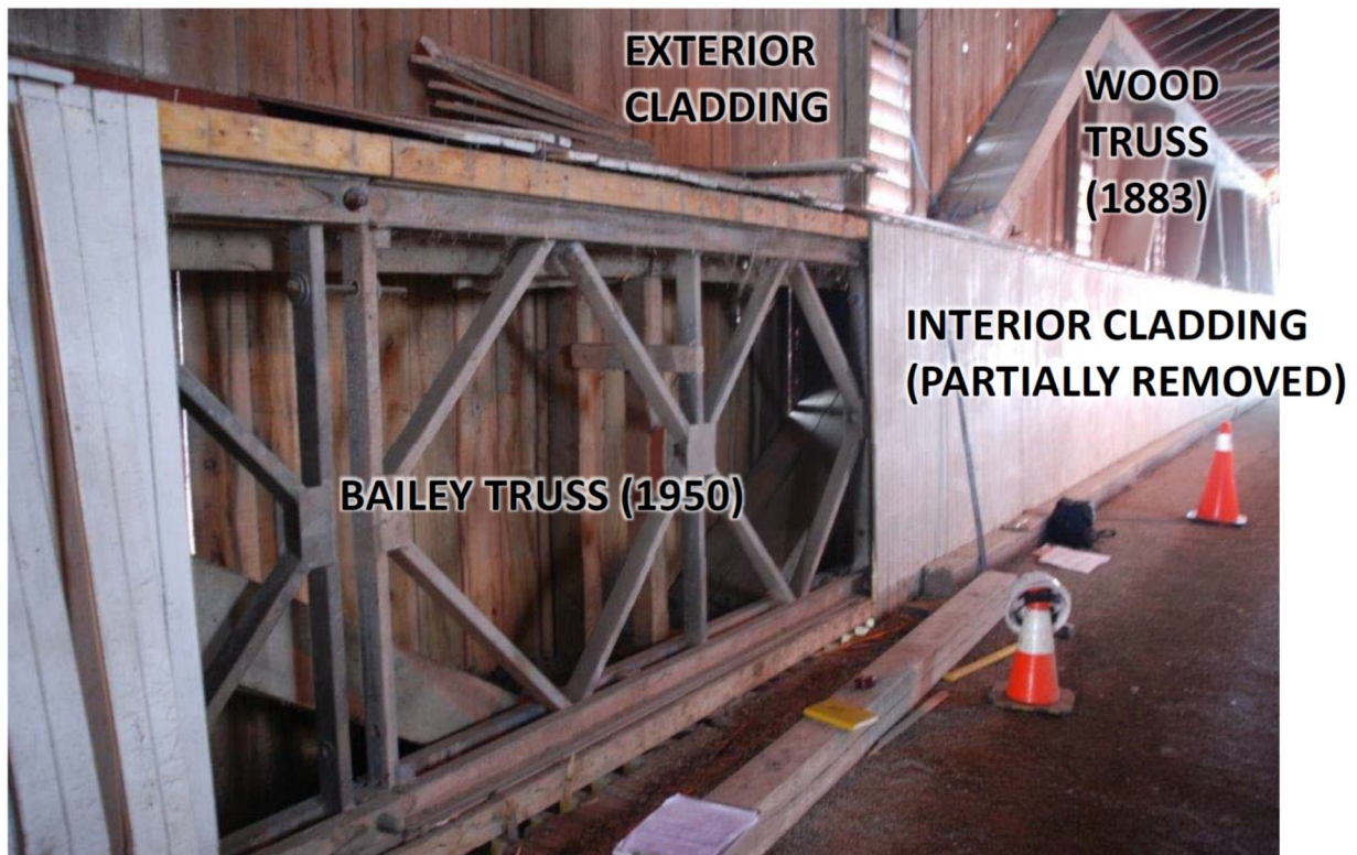
Figure B7: Interior View of Bailey Truss
