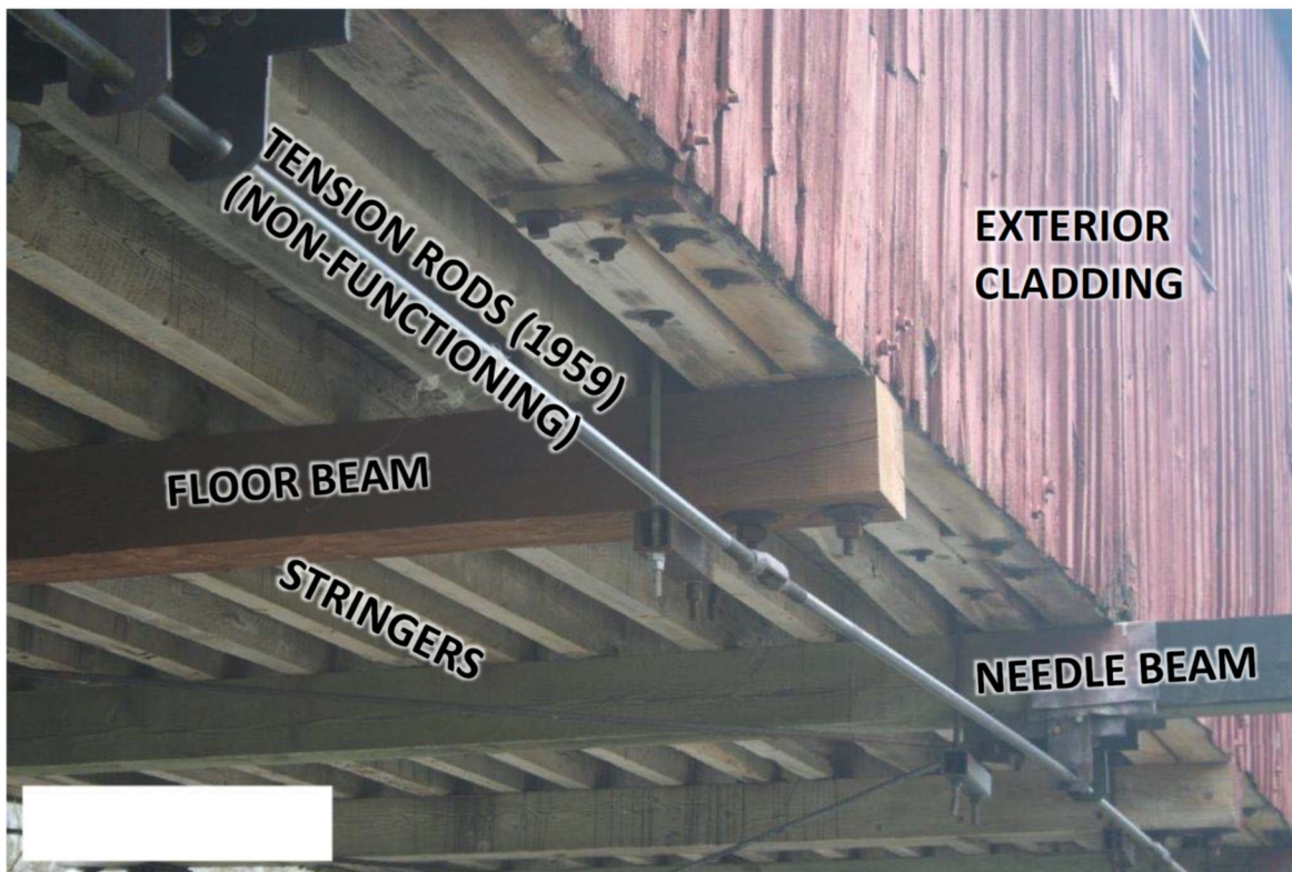
Figure B3: Exterior View
