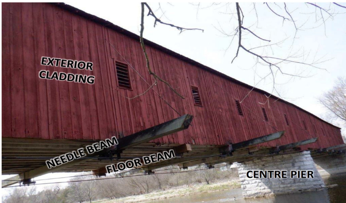
Figure B2: Exterior View
