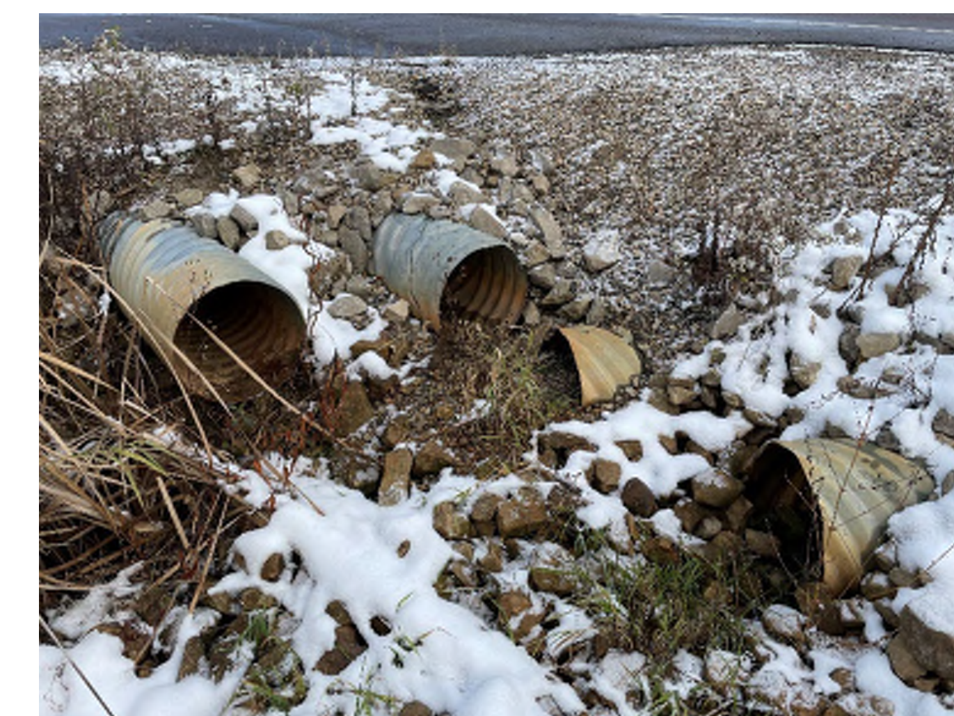
Outlet of Twin Culvert Set #1 (right) and inlet of Twin Culvert Set #2 (left)
