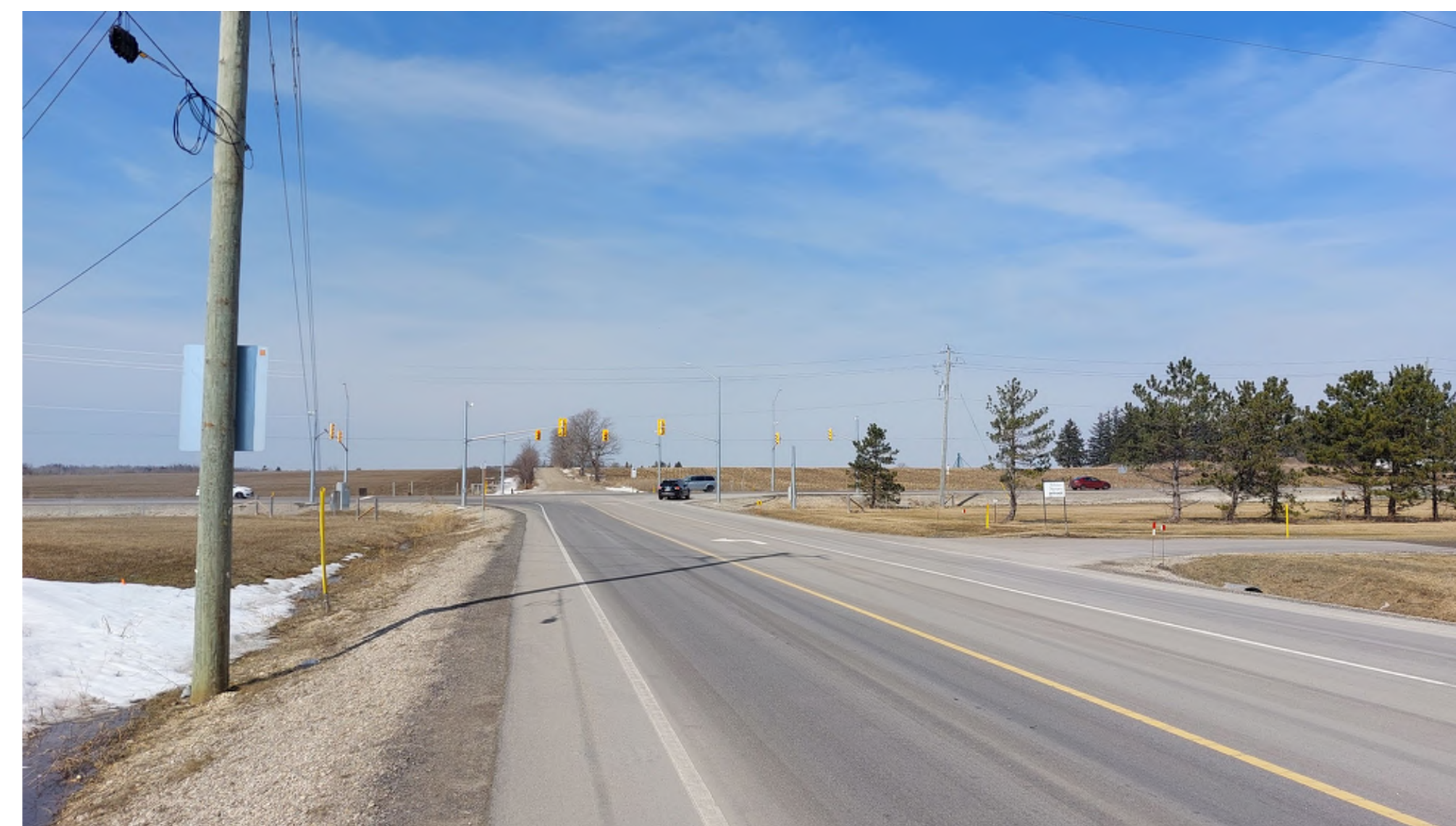
Greenhouse Road at Highway 7 (Victoria Street North)
