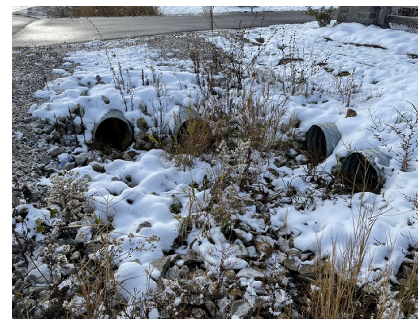
Outlet of Twin Culvert Set #2 (left) and inlet of Twin Culvert Set #3 (right)
