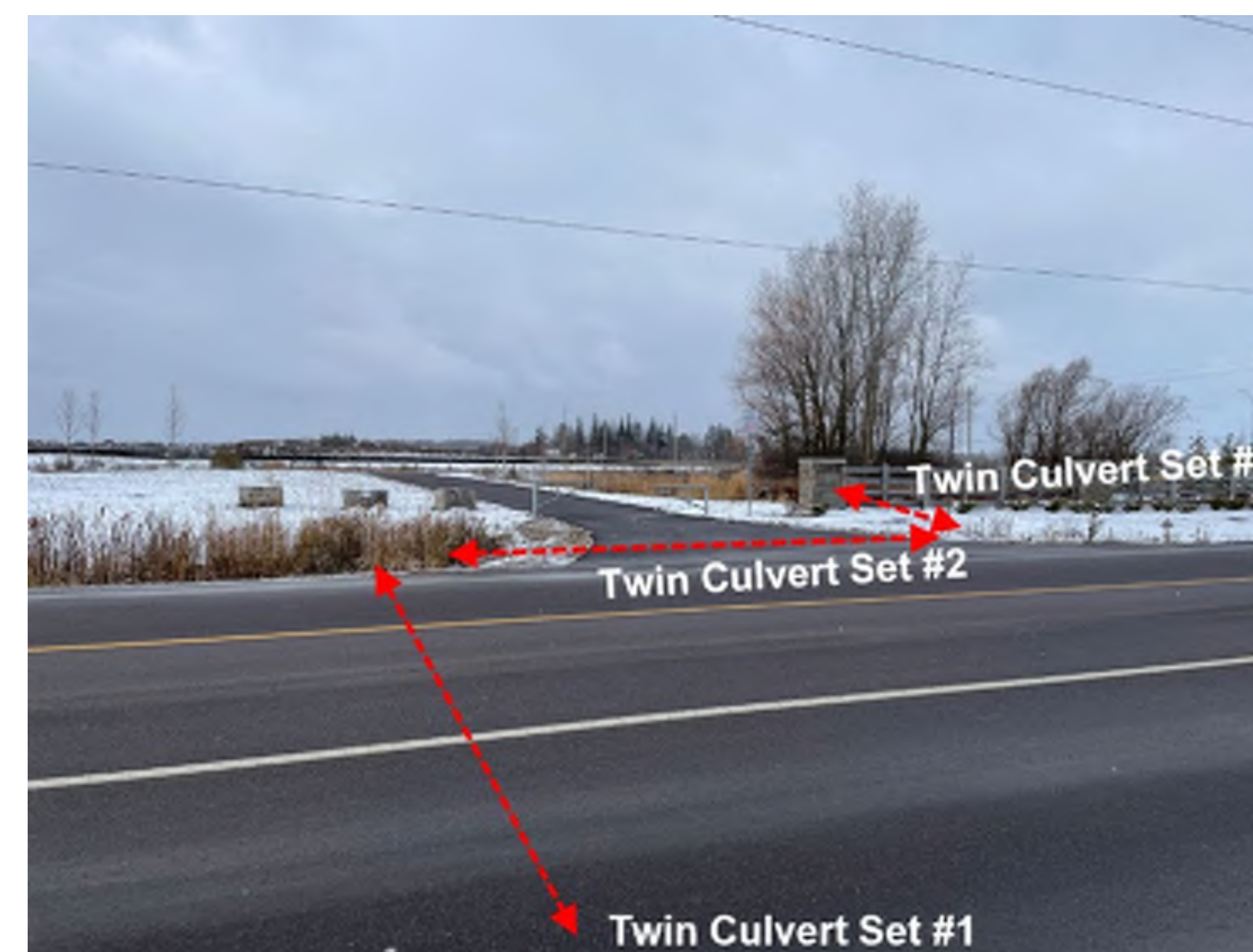
Crossing HC-East-Trib 1 – location of the three sets of twin culverts close to the intersection between Greenhouse Road and Highway 7 (Victoria Street North)
