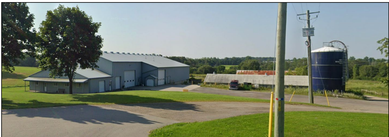
Figure 2: Existing Buildings and Accessories on 51-55 Hawkesville Road (Source: Google Maps)
