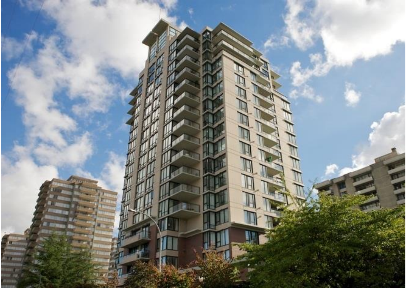
Example of high-rise residential development
