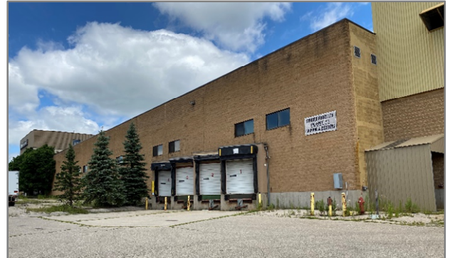
Building A, Warehouse and Distribution
