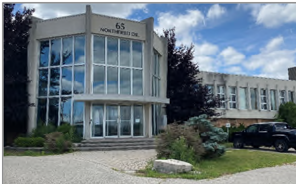
Building A, Administrative Offices
