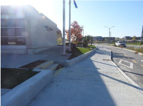
Example of a sidewalk
