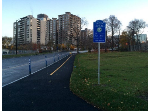
Example of a surface upgrade
