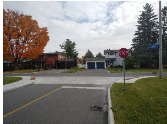
Example of a raised crosswalk
