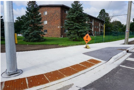
Example of a tactile attention indicator
