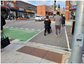
Shortened pedestrian crossing distances and the addition of accessible tactile walking surface indicators were included in the scope of construction for the downtown cycling grid. A study to add a new crossing at King and Eby Streets found that current sightlines will not be adequate to ensure proper visibility of crossing pedestrians. A new pedestrian crossing is recommended when a street reconstruction opportunity arises in the future.
