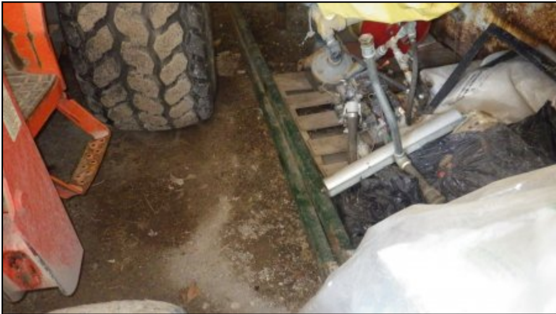
Staining observed within the Maintenance Shed at 100 Wilmot Line.
