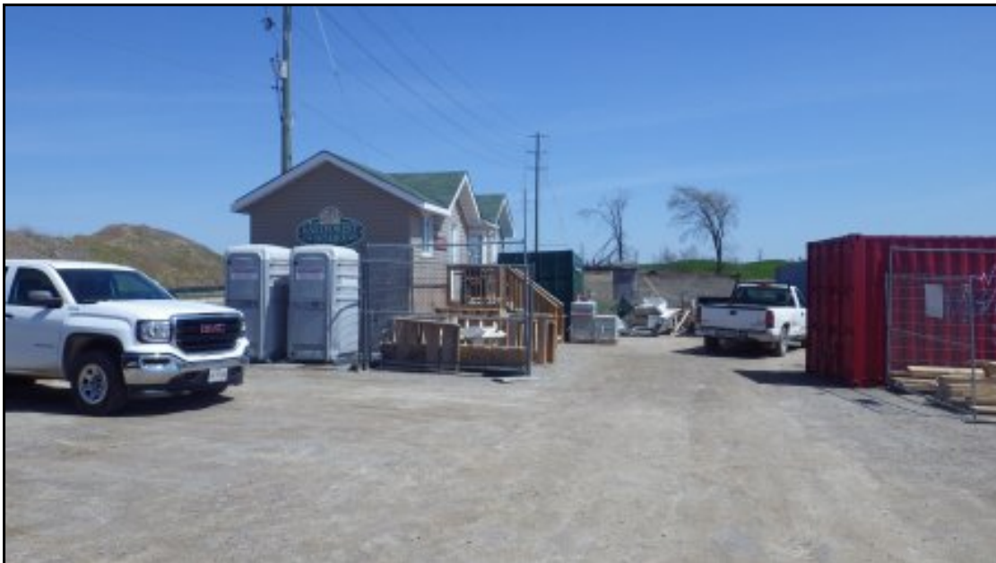
Construction Office at 250 Wilmot Line, facing north.
