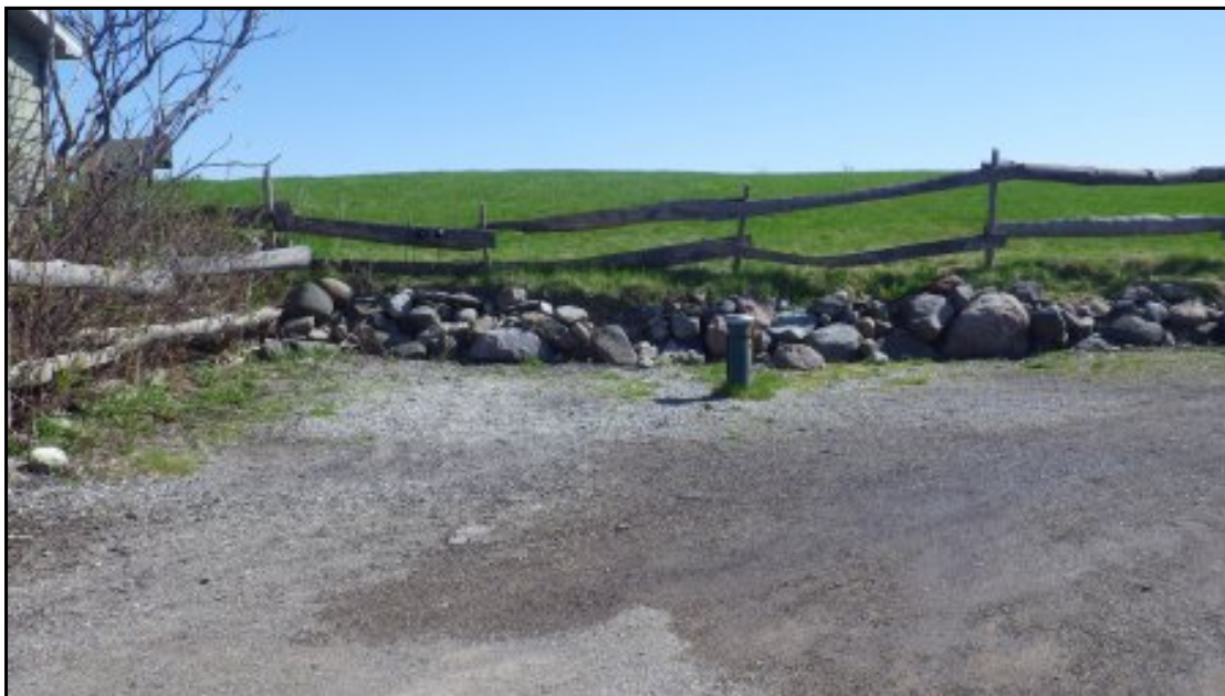
Water supply well situated southeast of the Driving Range Shed at 100 Wilmot Line, facing east.
