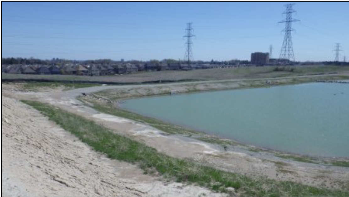
Stormwater management pond situated on the eastern edge of 100 Wilmot Line, facing east.
