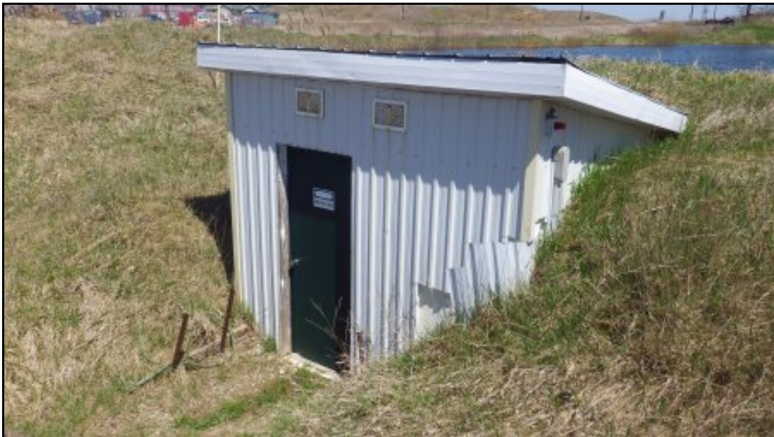
Pump House Shed at 100 Wilmot Line, facing north.
