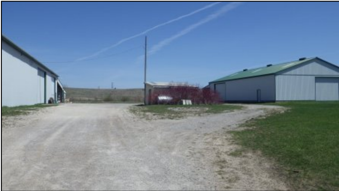
Observed ASTs at 50 Wilmot Line, facing east.
