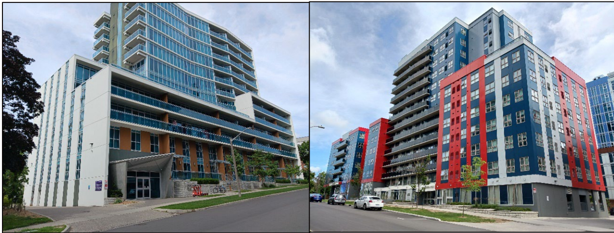
Figure 3-4 Neighbouring Apartment Building responses to topography with 255 Sunview Street (left) and 258B Sunview Street (right) (Source: Arcadis)
