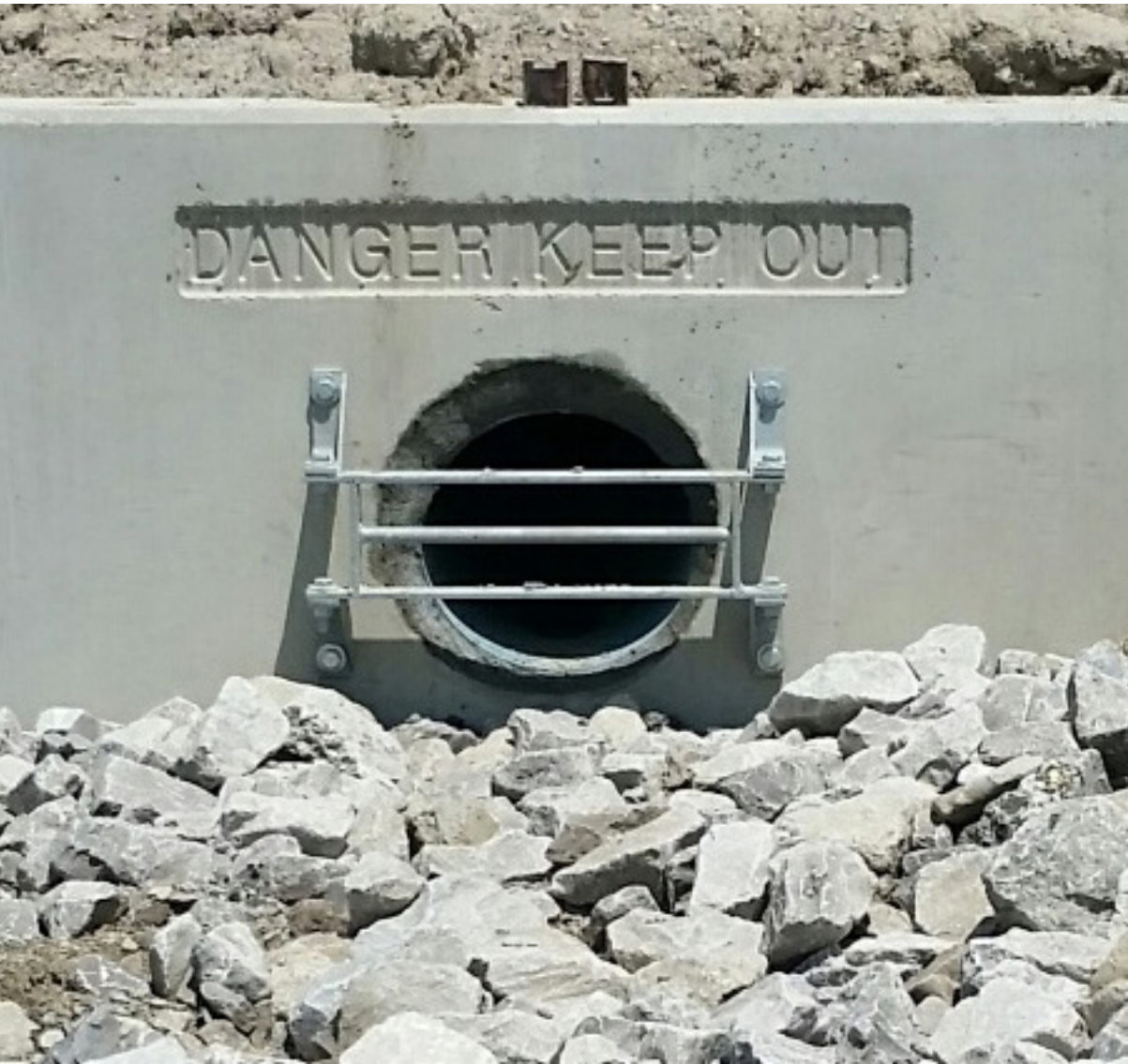
5 Sewer Safety Grate
