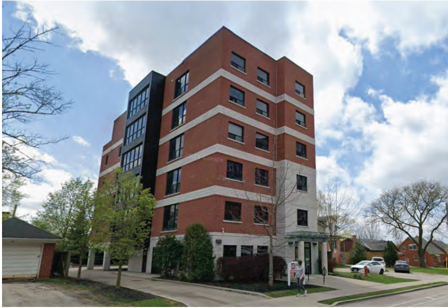
Figure 2.5 - 6-storey residential building immediately east of the Site
