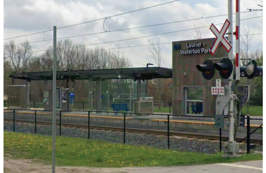
Figure 2.8 - Laurier-Waterloo Park ION LTR station
