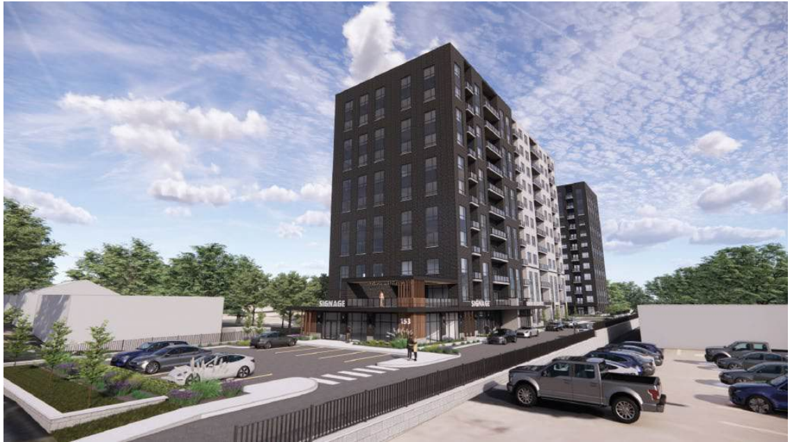
Image 3: View of Building A from Union Street East
