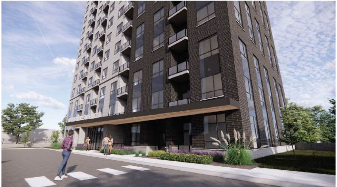
Image 7: View of Building B from Interior of Site
