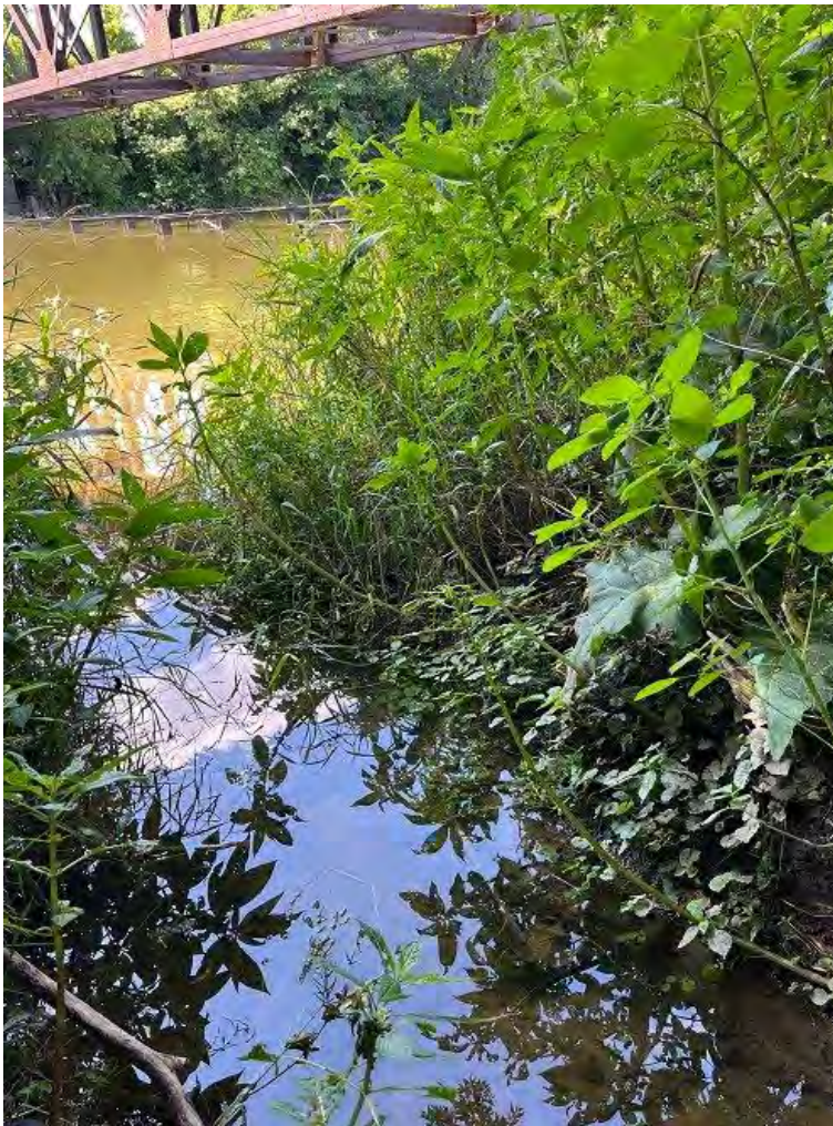
Figure 4. On-site drainage swale outlet connecting to Conestogo River during high flow, facing downstream from on-site drainage swale
