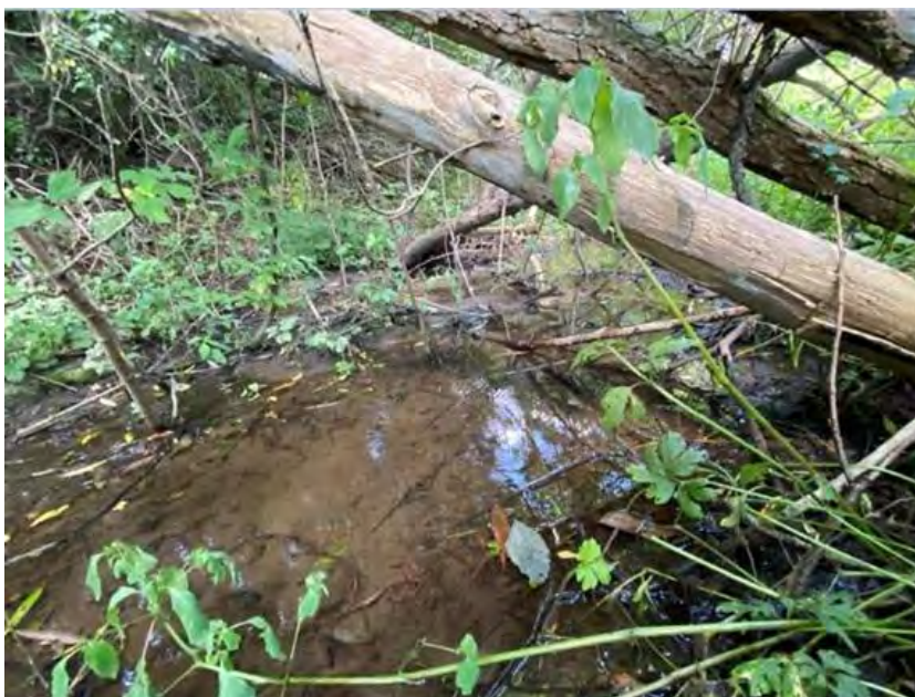
Figure 8. Pooling of drainage swale adjacent to the floodplain within approximately 10m of the drainage pipe, facing upstream
