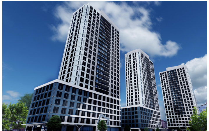
FIGURE 24: TOWER VIEW - LOOKING WEST
