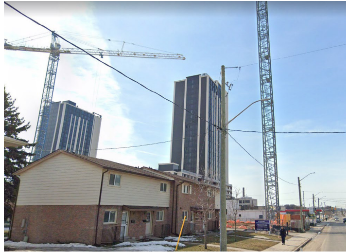
FIGURE 4: COLUMBIA STREET WEST - LOOKING WEST AT SUBJECT SITE
