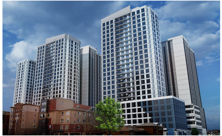
FIGURE 26: TOWER VIEW - LOOKING EAST
