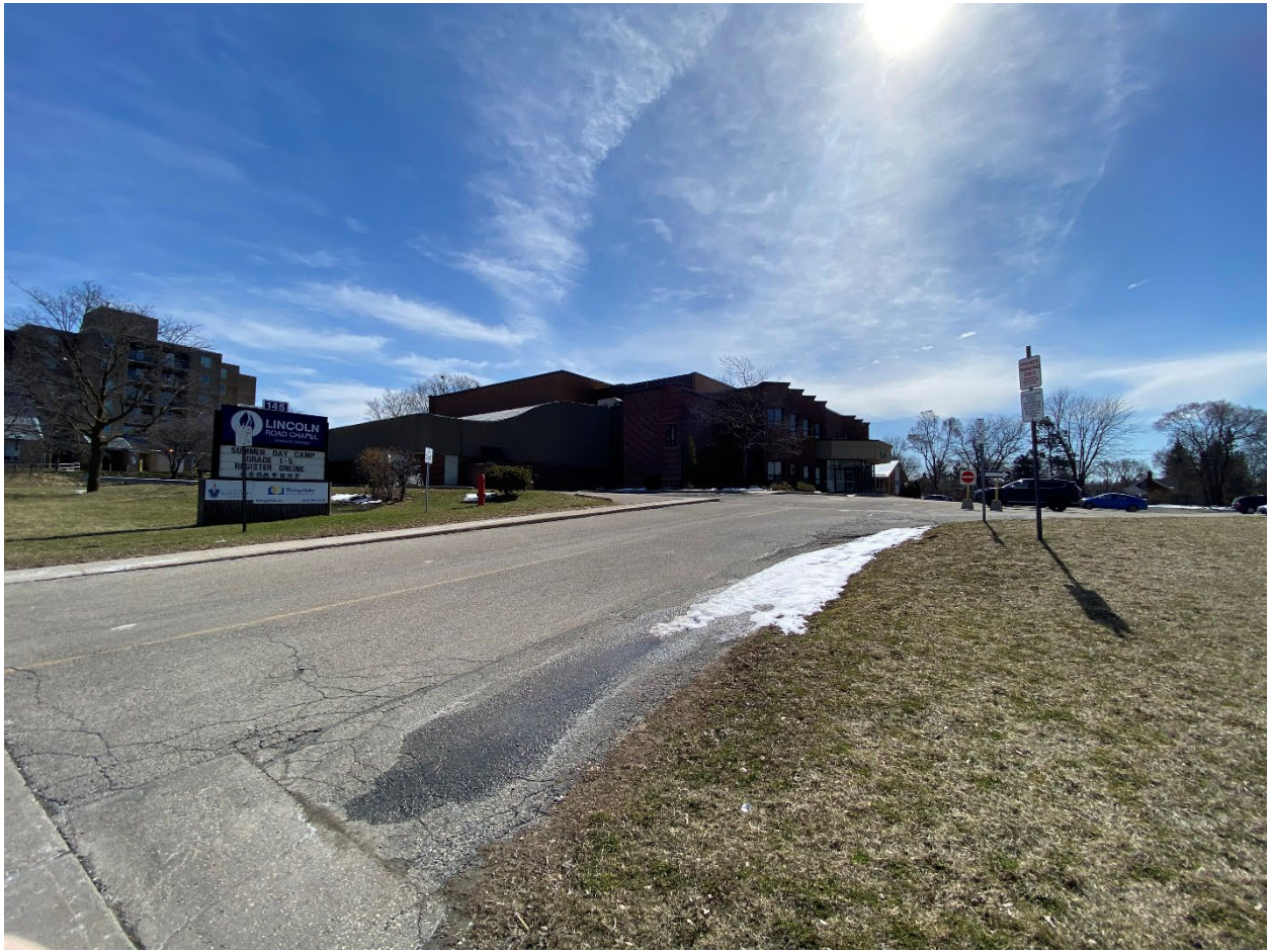
Figure 6: Existing Church Building, Viewed from Lincoln Road
