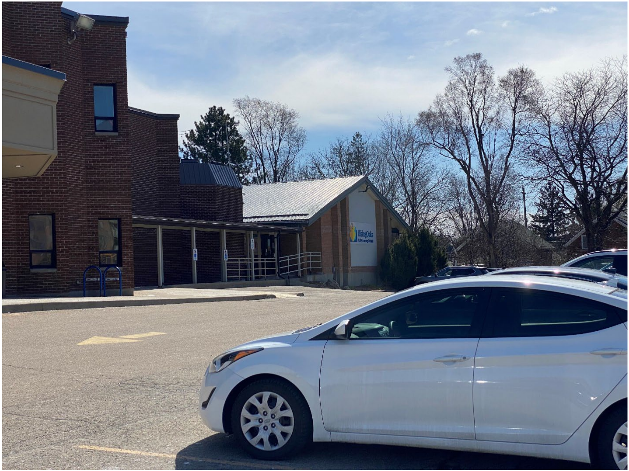
Figure 8: Existing Daycare Building
