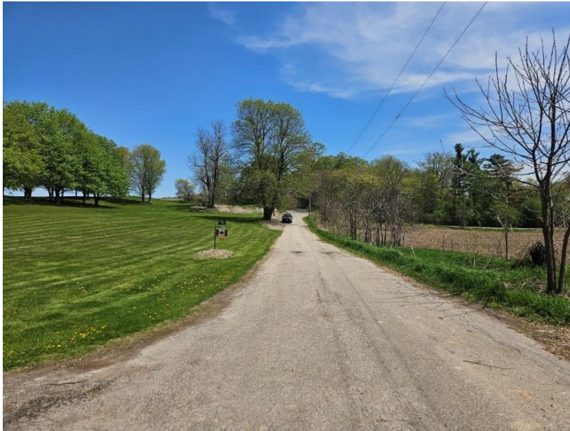
Figure 4: Stauffer Drive looking east from Reidel Drive, showing its narrow two lanes and no shoulders (A.S.I., 2025).
