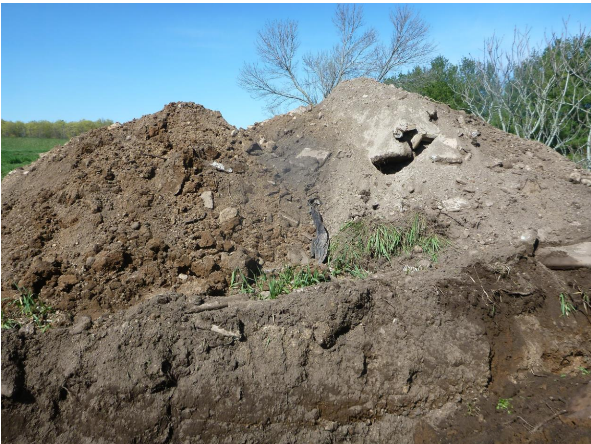
Photograph 2: View of construction debris in excavated material of TP1
