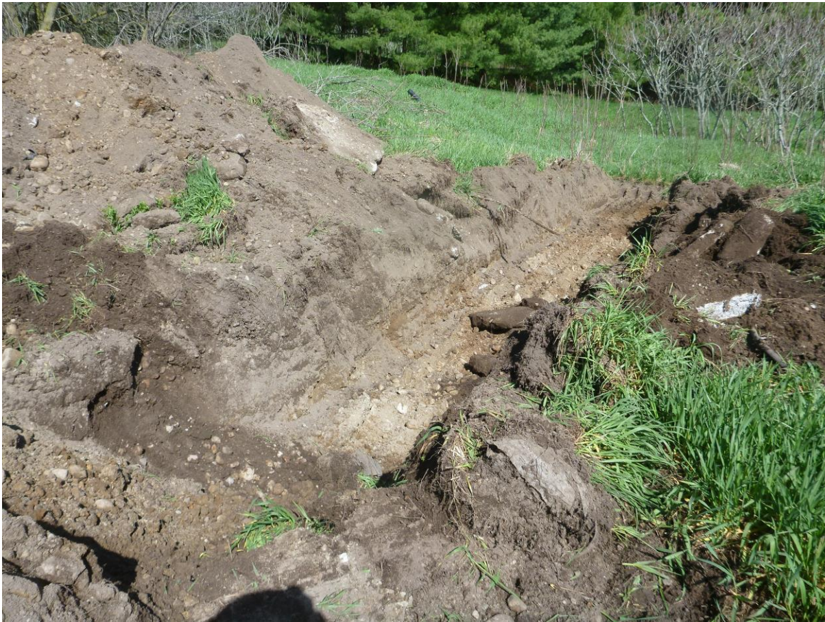
Photograph 3: View of test pit TP2
