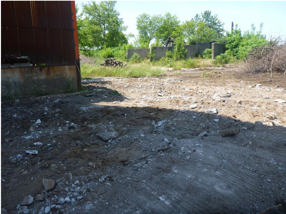
Photograph 3: Excavation of waste oil impacted concrete pad and soils.
