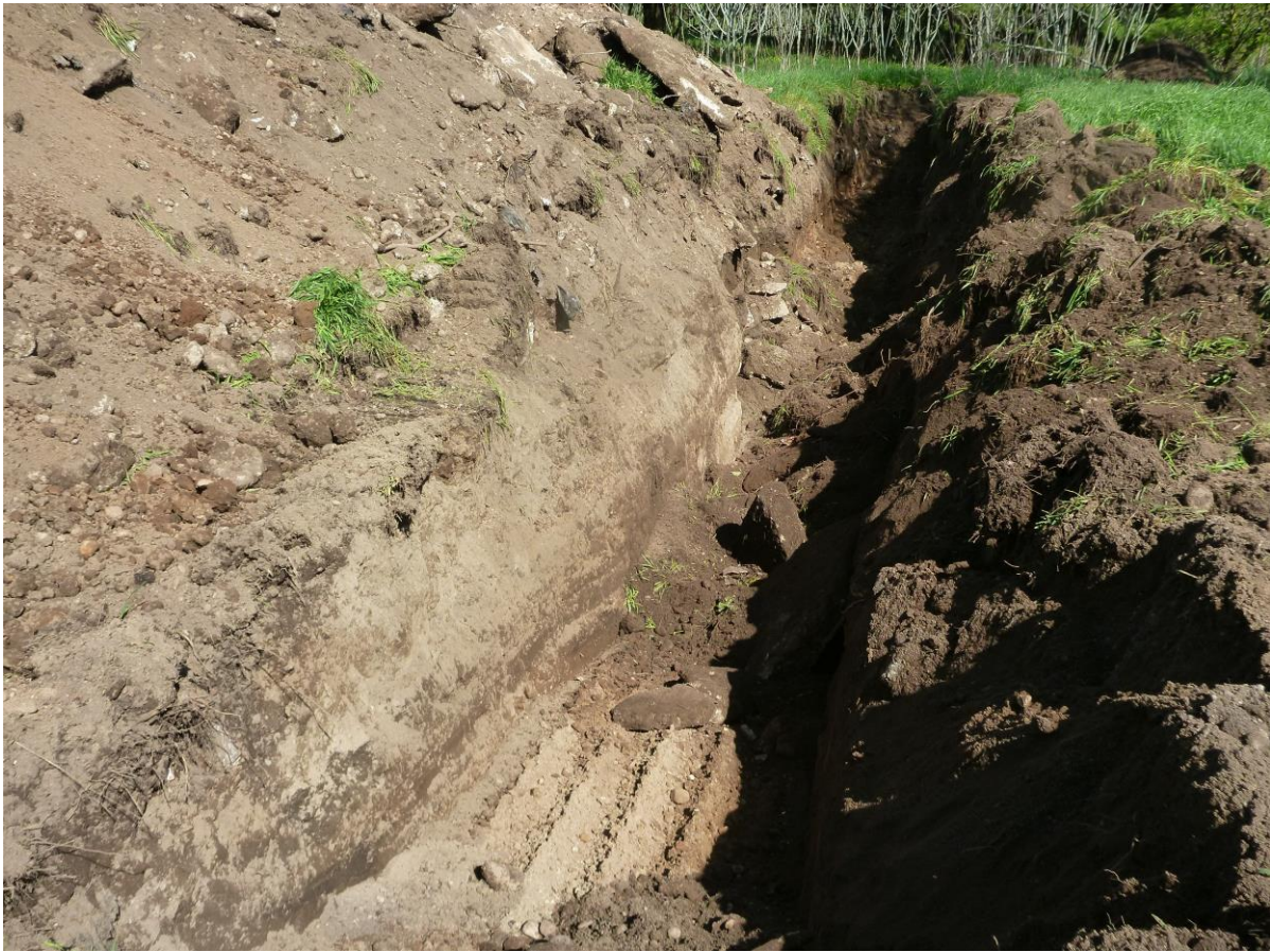
Photograph 5: View of test pit TP3
