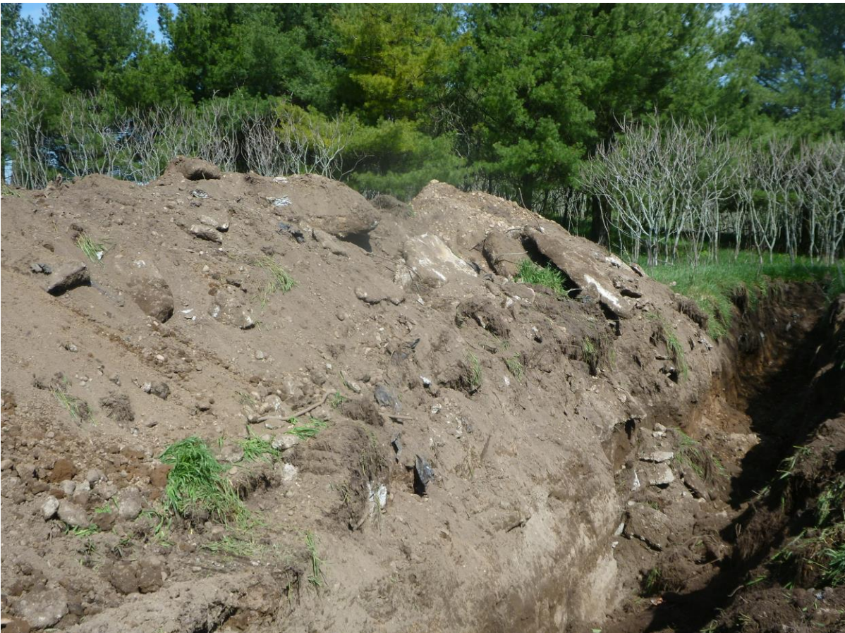
Photograph 6: View of construction debris in excavated fill material of TP3
