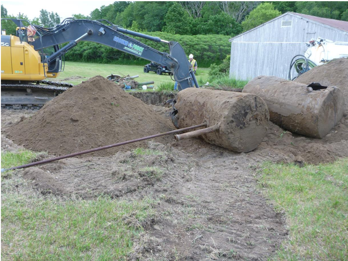
Photograph 2: Excavation of USTs and hydrocarbon impacted soils.
