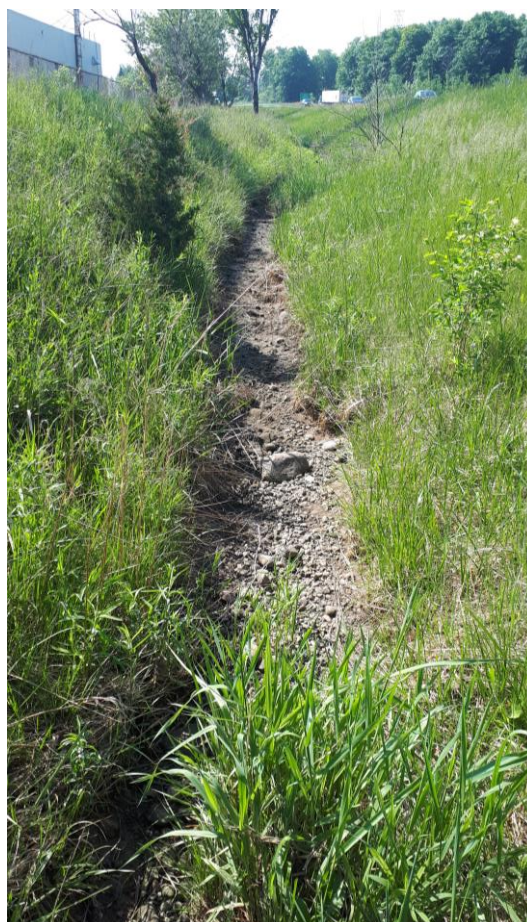
Figure 3. Drainage ditch along Hwy. 85, facing southeast (June 5, 2020).
