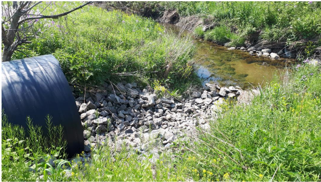
Figure 4. Culvert #3 outlet to Forwell Creek (June 5, 2020).
