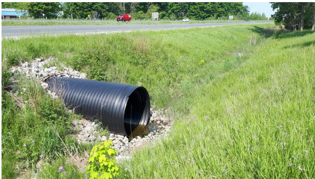
Figure 2. Drainage ditch at inlet to culvert #3, facing northwest (June 5, 2020).
