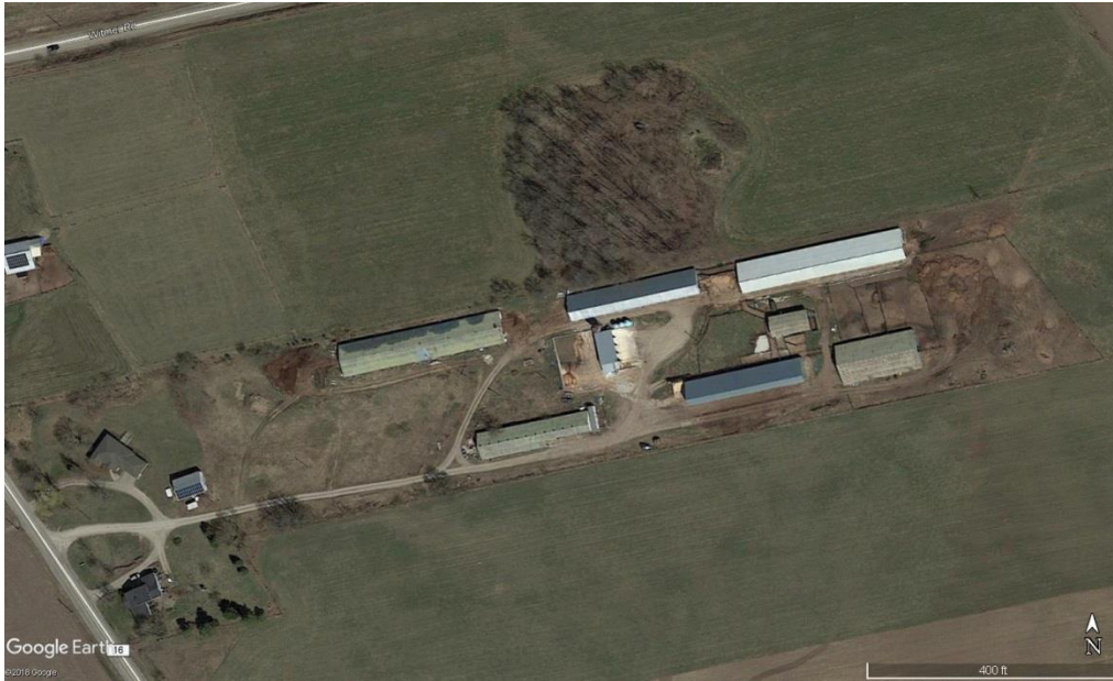
Agricultural Facility #4, #5, #6, #7, #8 and #9
