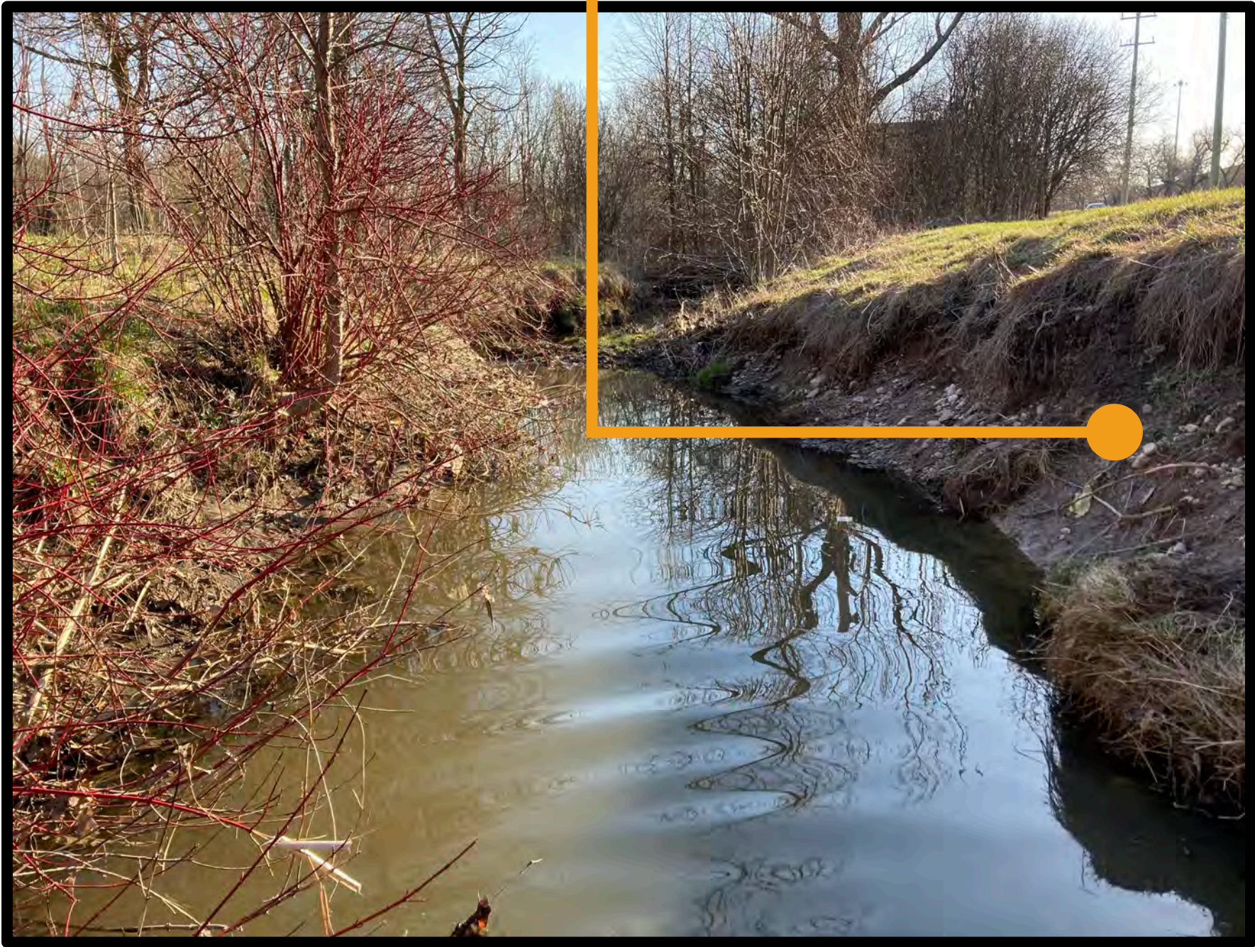
Eroding banks, exposed bare soil
