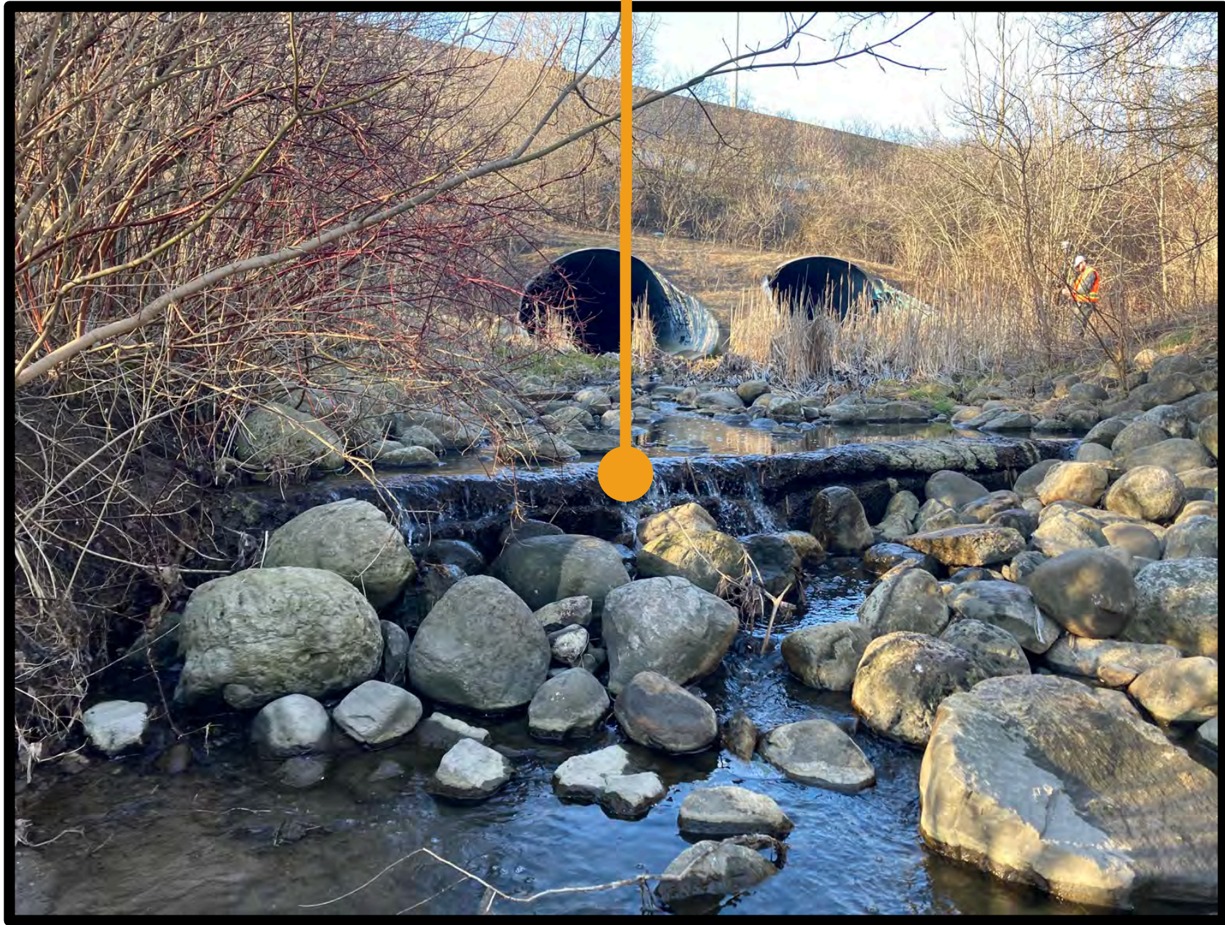
Exposed sanitary pipe (concrete-encased)
