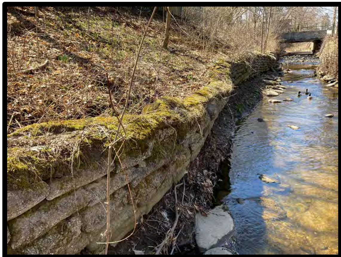
Slumping Retaining Wall
