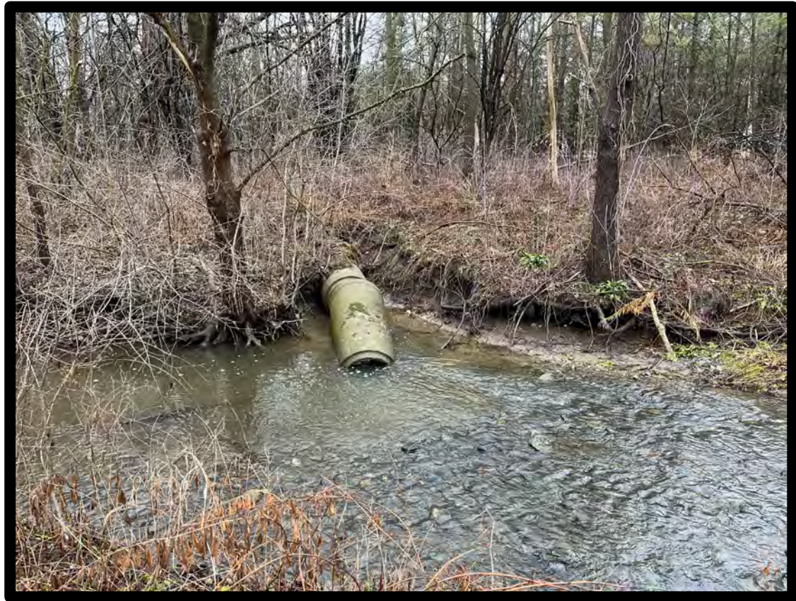
Failed Stormwater Outlet
