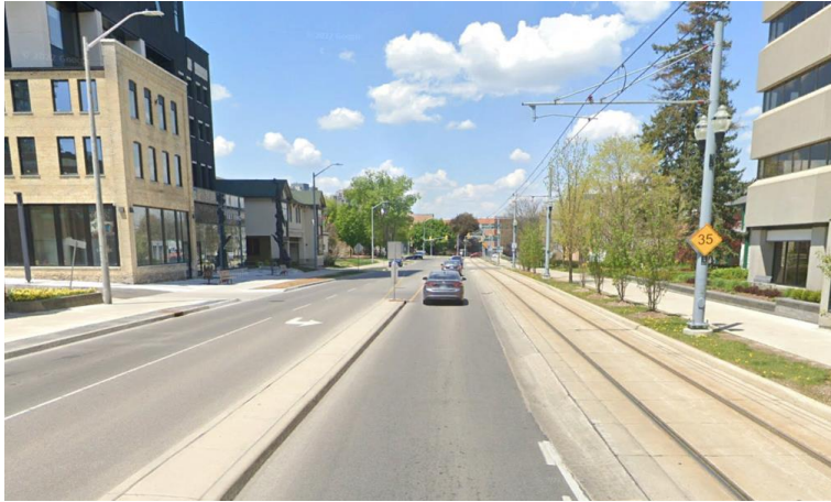
Figure 2a: Looking northwest along King Street South
