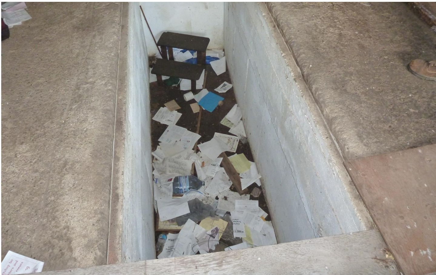
Photograph 9: View of the floor trench/mechanics pit within the derelict maintenance shop building.
