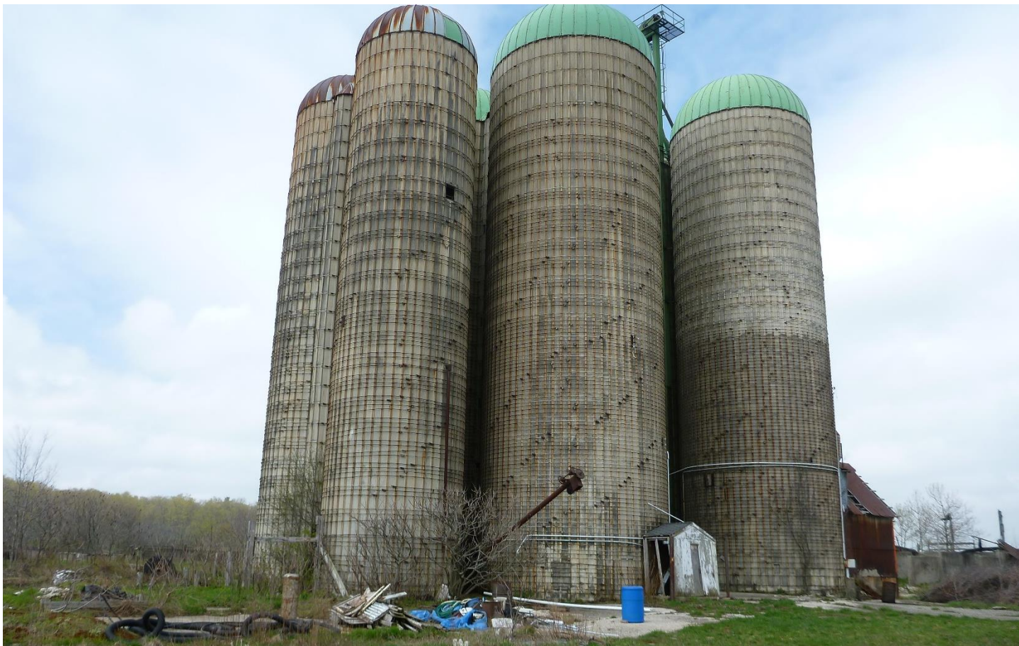
Photograph 5: View of the silos on the south end of the Site.
