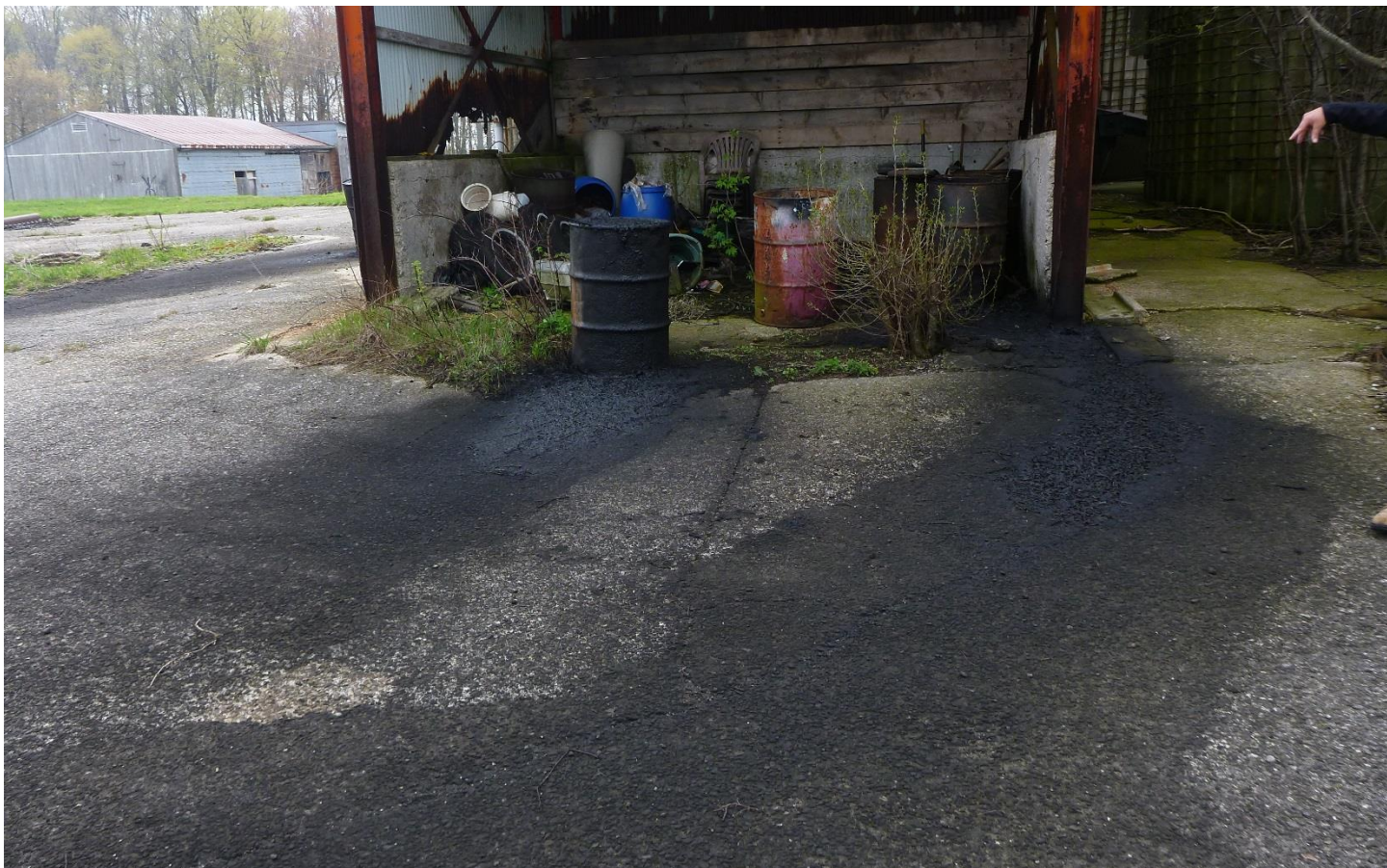
Photograph 6: View of the corroded waste oil drums adjacent to the silos. Ground surface is stained with leaked oil.
