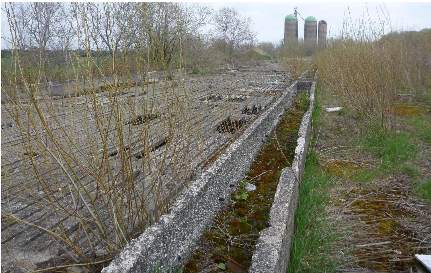
Photograph 4: View of the demolished cattle pens on the south end of the Site.
