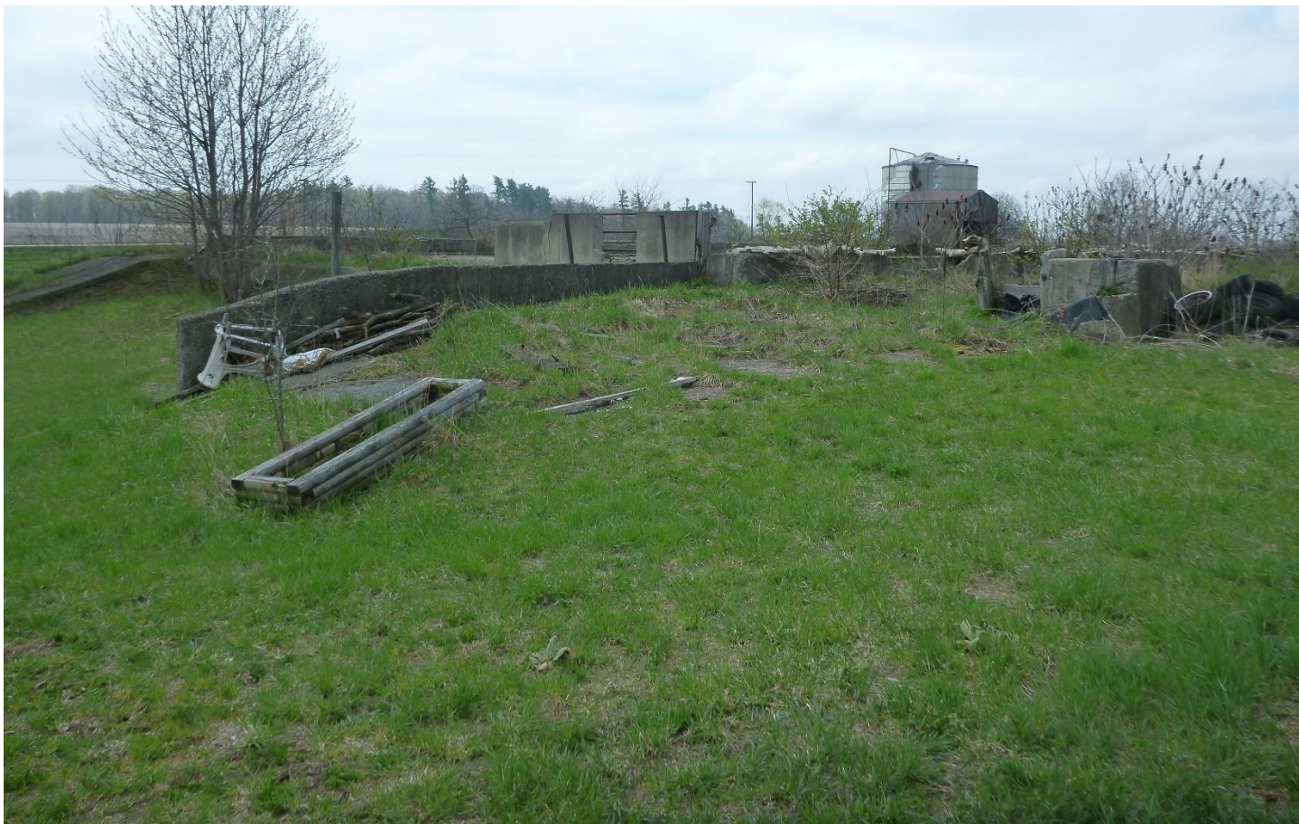
Photograph 1: View of the front (south end) of the Site with derelict commercial farm structures.
