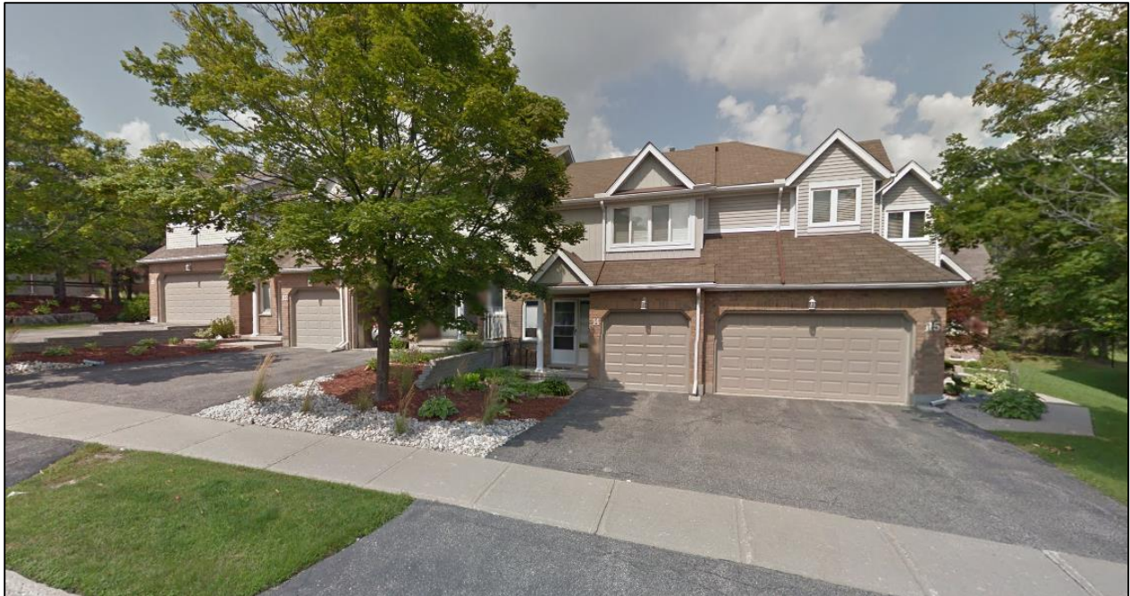
Figure 9: Northern view of townhouses at 522 Beechwood Drive (Google, August 2015)
