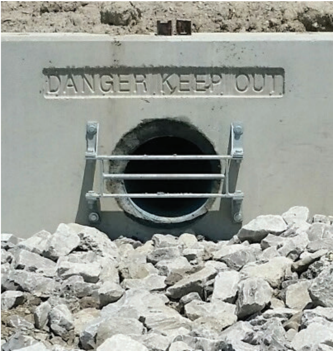
Sewer Safety Grate
