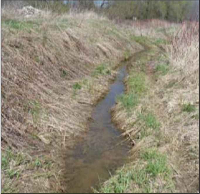
Water draining out of agricultural field drain into Unit 8— May 3, 2020
