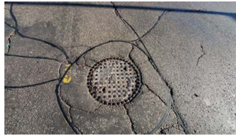
Subsurface Utility Investigation
