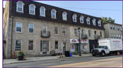
Aerial view of 22 Queen St W.
