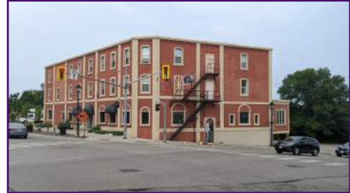
Aerial view of 7 Queen St W.
