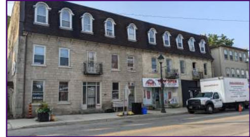
Aerial view of 16 Queen St W.
