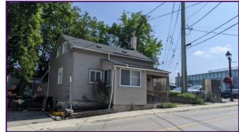
Aerial view of 9 Adam St.
