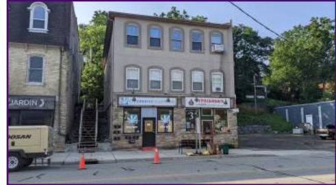
Aerial view of 26 Queen St W.
