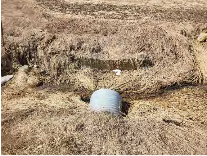
Photo 31. Culvert C4 upstream of New Jerusalem Road.
