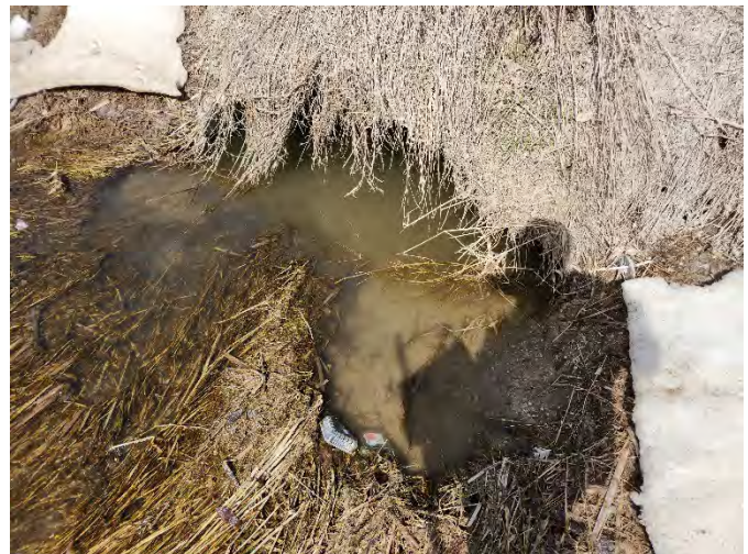
Photo 36. Culvert C5 downstream of Scotch Line Road.
