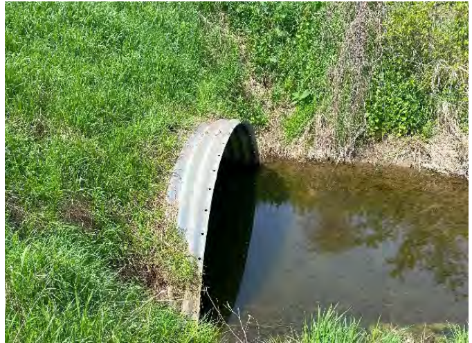
Photo 6. Culvert C1 downstream of South Field Road.
