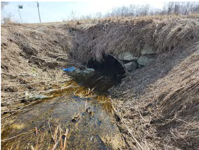
Photo 35. Culvert C5 upstream of Scotch Line Road.
