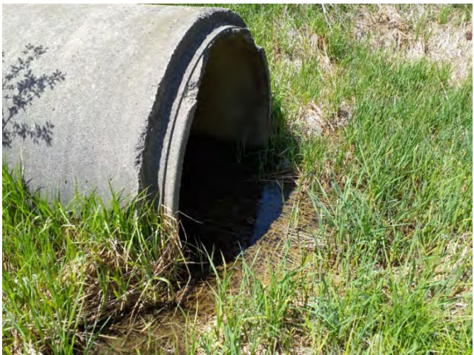
Photo 23. Culvert C2 upstream of South Field Road.
