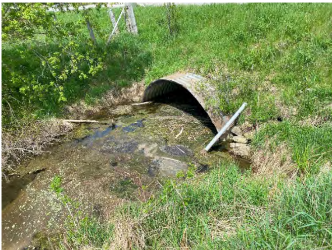
Photo 5. Culvert C1 upstream of South Field Road.
