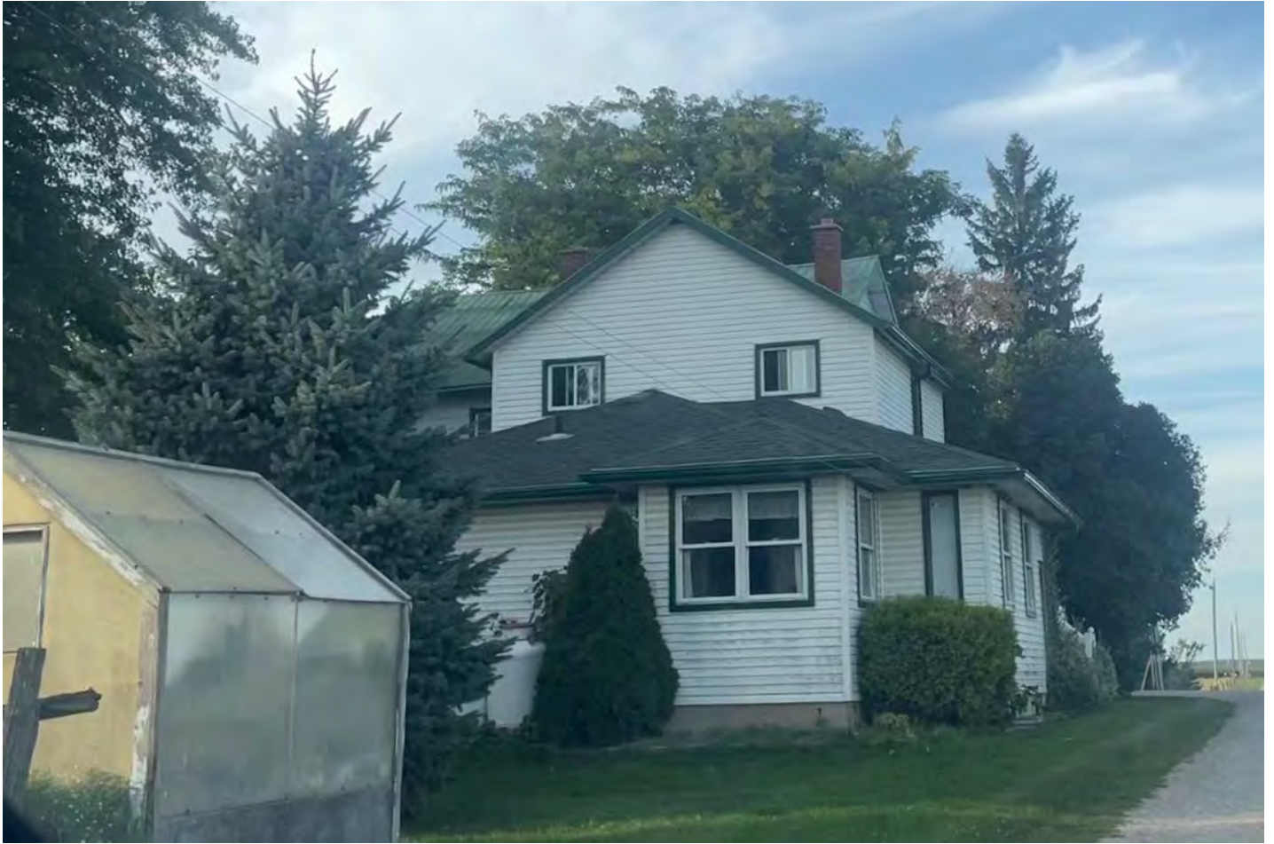
Photo 37. View of traditional chimneys on the current farmhouse that may provide habitat for Chimney Swift.
