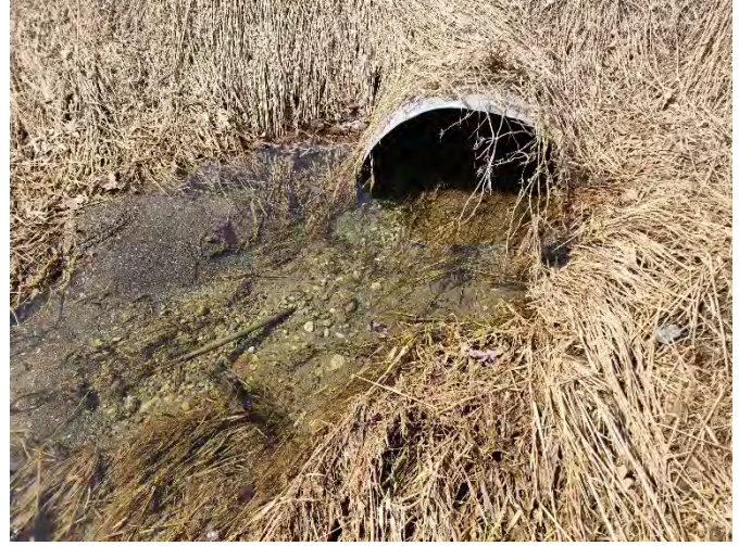
Photo 32. Culvert C4 downstream of New Jerusalem Road.
