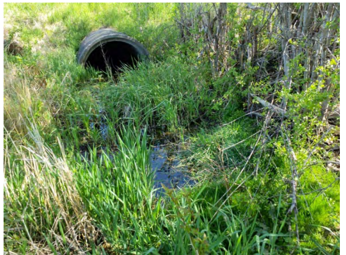
Photo 24. Culvert C2 downstream of South Field Road.
