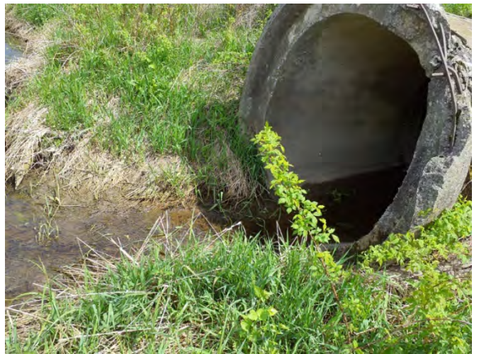
Photo 18. Culvert C3 downstream of railway.
