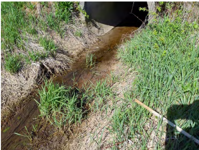
Photo 17. Culvert C3 upstream of railway.
