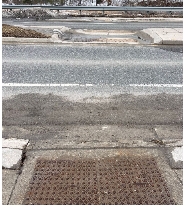
Figure 7: Existing Pedestrian Crossing
