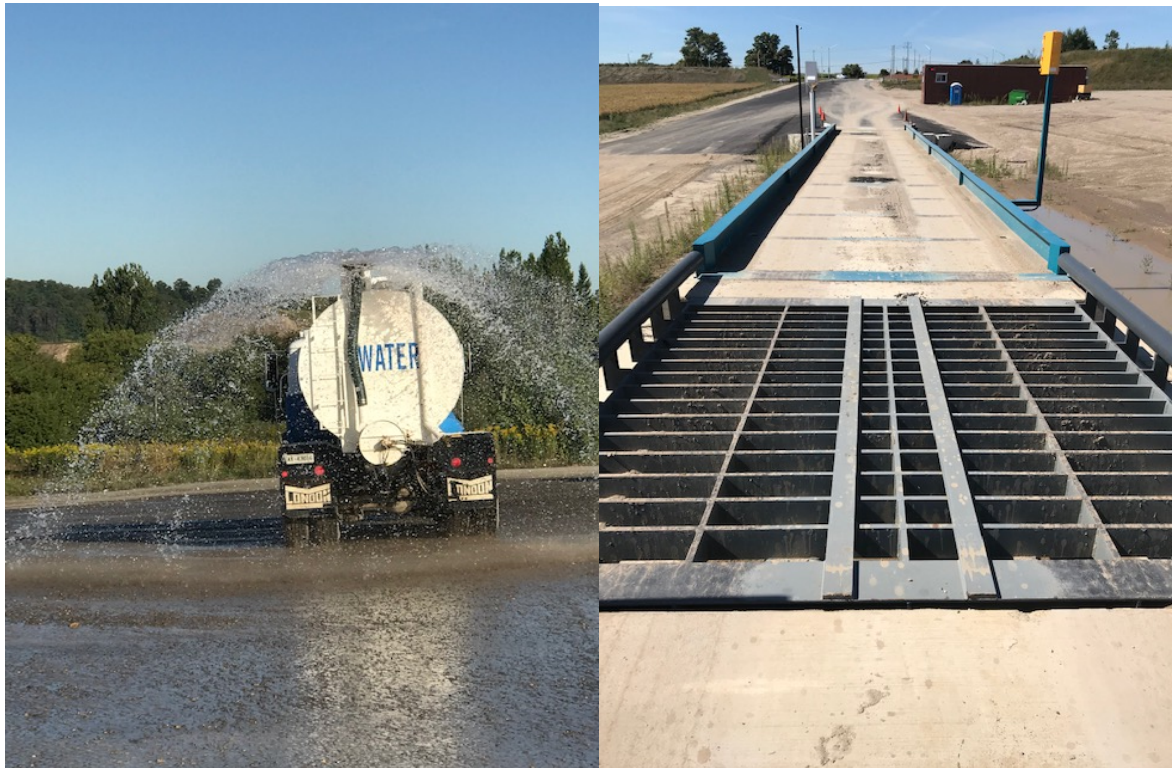
Figure 6.1 Water truck (left) and Grizzly screen (right)
