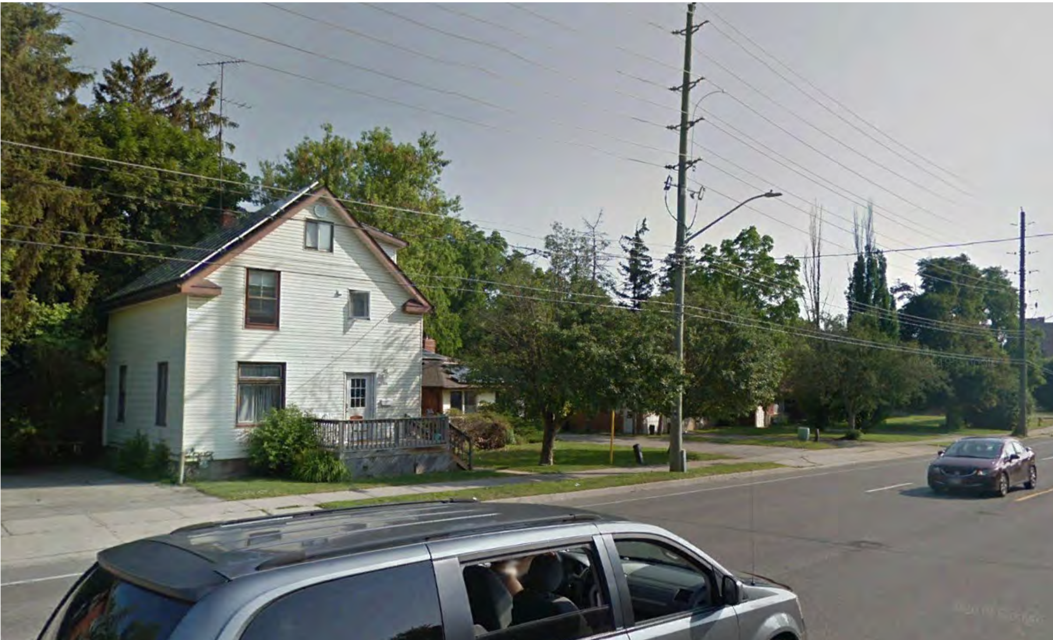
SITE CONTEXT / VIEW FROM ERB STREET WEST
